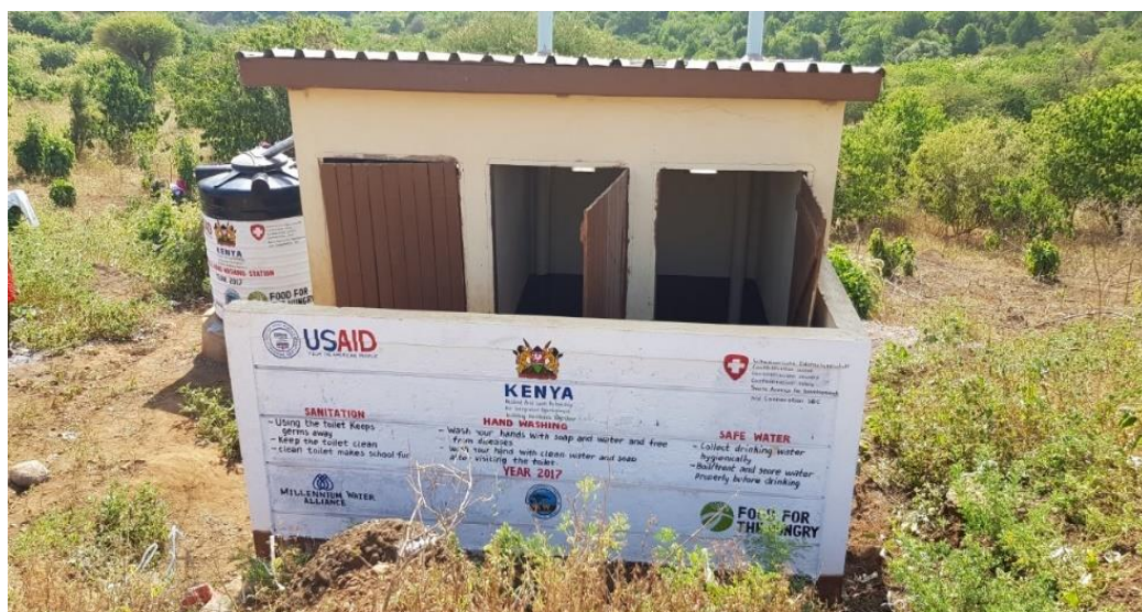
One of the 3-Door VIP latrines built through Kenya RAPID support
