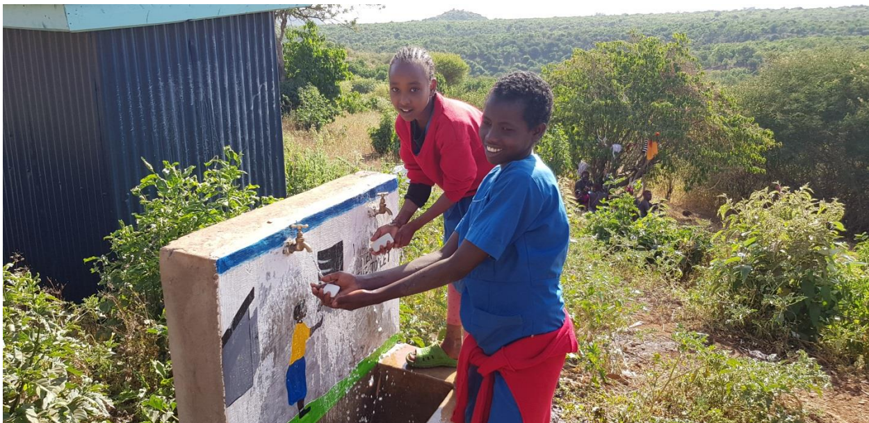
A hand washing point constructed at Ilpus Primary School under funding from Kenya RAPID program. Photo credit: Johnson Ng'ang'a
