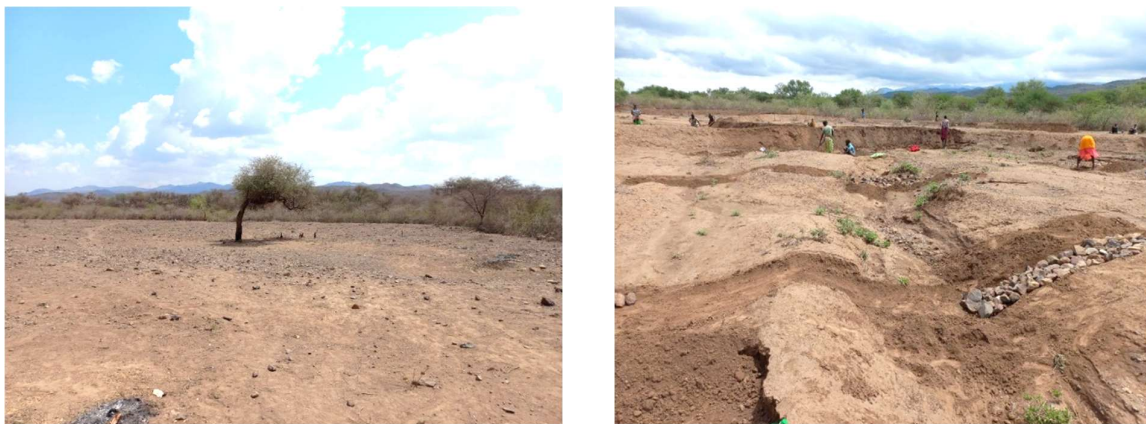
Left: A degraded field in Pelekech with minimal vegetation cover; Right: Construction of half-moon bunds to mitigate soil erosion and address gullies in Pelekech.
